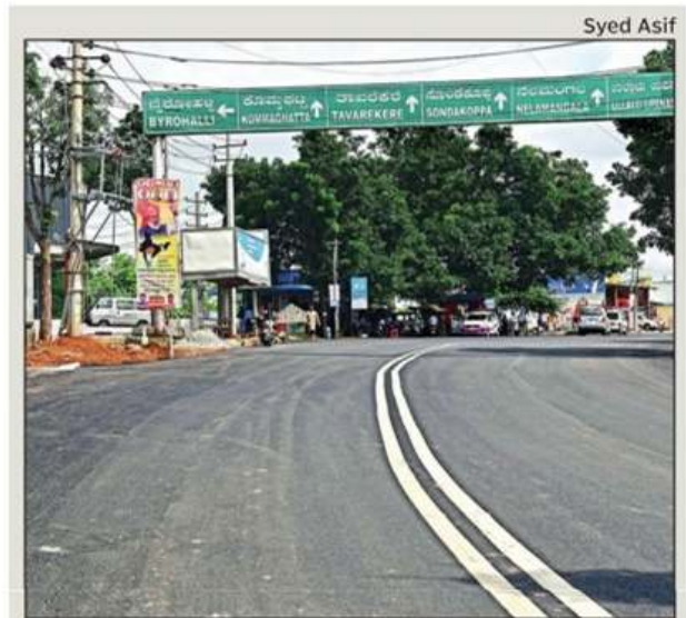
SMOOTH WORK: A road in Kammaghatta, Kengeri, that was asphalted ahead of PM Modi's visit
